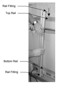
2. Secure Channel by tightening the top Rail Fitting (2) 10-32 x 3/4" OHMS & (1)10-32 x 3/4" PHMS.
