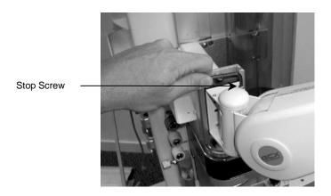
Note: For right side installation, install the VHM stop screw in opposite side hole on rear pivot bracket.
